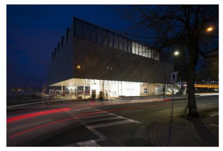
The striking new construction at the southern end of Lonsdale Avenue was designed by Patkau Architects as a two-floor building. Above the generously glazed ground floor with foyer, shop and café area at street level is the gallery floor, clad with stainless steel shingles and benefiting from daylight through the bands of windows of the sawtooth roofs.
